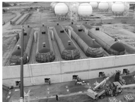
Fig. 2 Completion of construction of propylene horizontal tanks in LPG storage area (Source: [24])
